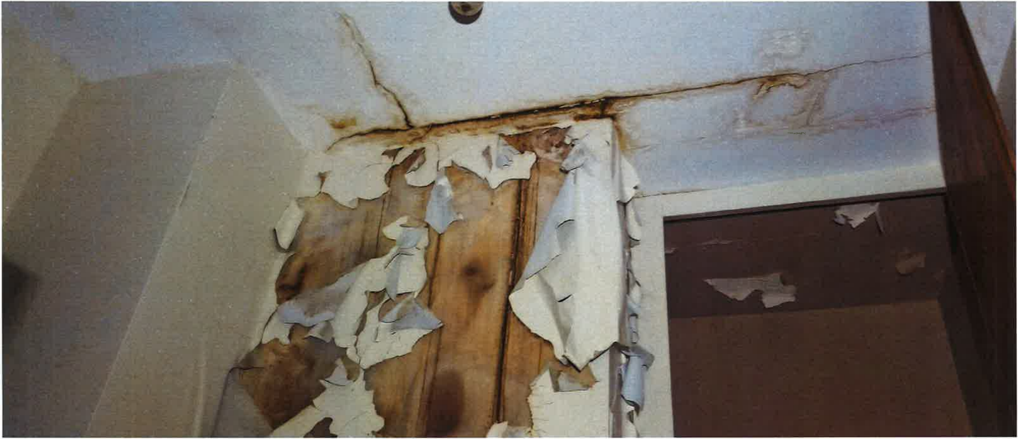
Evidence of Moisture Damage
