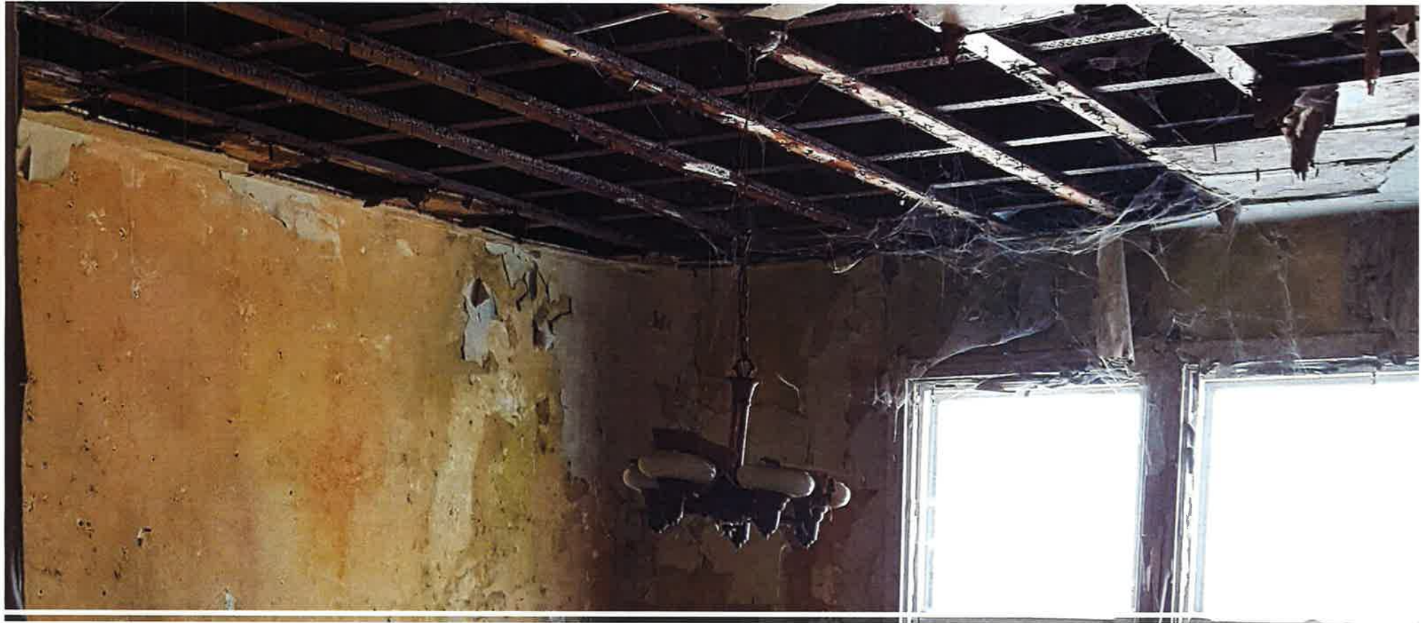
Deteriorated Ceilings & Wall Finishes (Typical)
